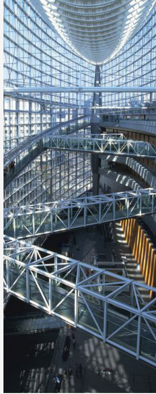
Steel Structure Engineering
